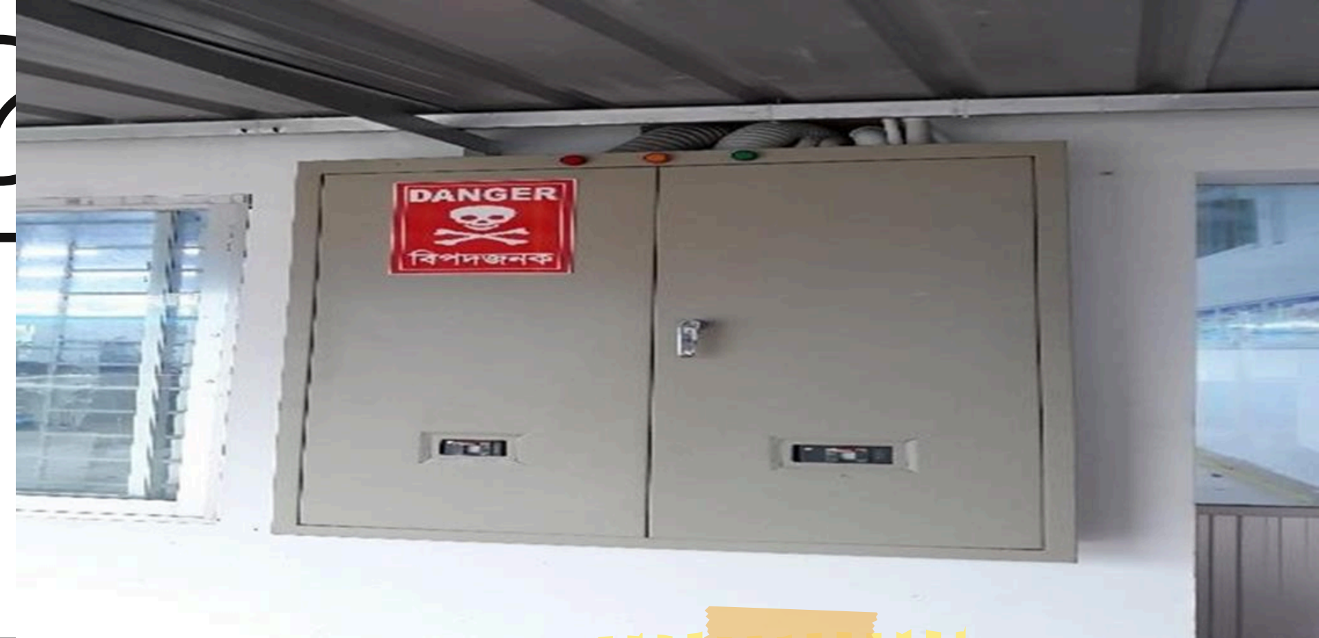
Electrical Main Switch Board
